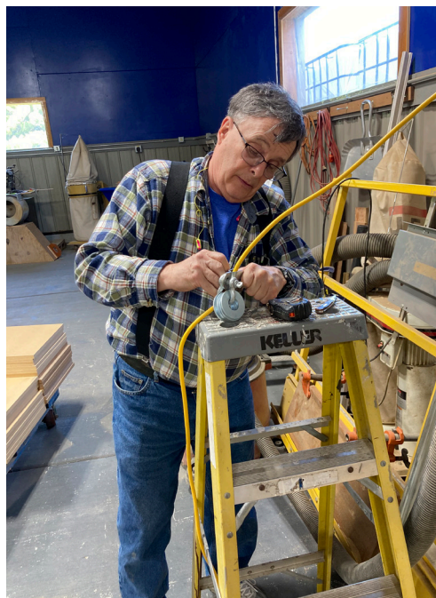
Mike Prince works on the repair.
